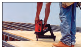
Plywood attachment—using TrakFast plywood to steel pin
