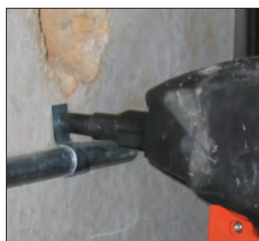
12HSMPO34 clip assembly used to secure conduit
